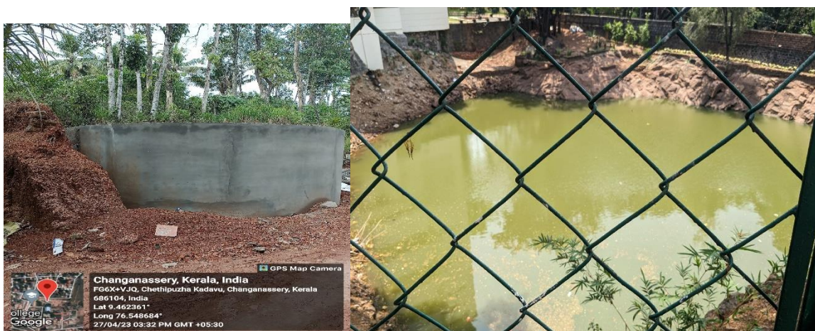
Figure 13 RAIN WATER RECHARGING FOR BOREWELL AND POND
